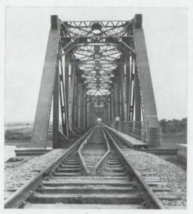
WARDHA RILWAY BRIDGE 7 SPANS, 200 FT THRO' TYPE RIVETTED
